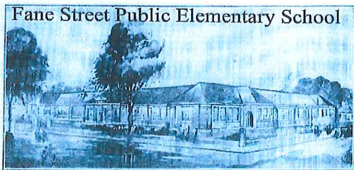
FANE STREET PUBLIC ELEMENTARY SCHOOL—NEW SCHOOL ON TWO-ACRE SITE TO ACCOMMODATE 200 PUPILS IN TWENTY CLASSROOMS, WITH LARGE ASSEMBLY HALL, SCIENCE LABORATORY, ART, COOKERY, AND WOODWORK ROOMS. BUILDING IS OF THE SINGLE-STORY TYPE, WITH CLASSROOMS ROUND TWO QUADRANGLES, WHICH ARE DIVIDED BY THE ASSEMBLY HALL. MESSRS. H. & J. MARTIN ARE CONTRACTORS FOR THE WORK, WHICH IS AT PRESENT WELL IN HAND. MR. F. S. WILSHIRE, A.R.T.A., F.R.S.E., THE EDUCATION ARCHITECT, IS RESPONSIBLE FOR SCHOOL BUILDINGS UNDER THE RELEASED EDUCATION AUTHORITY.
